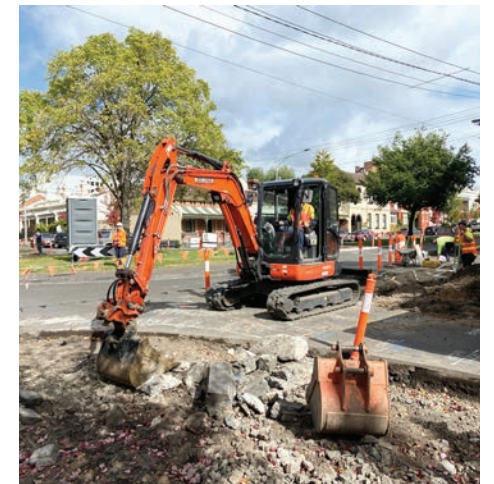
▲ Works are under way in East Melbourne.
