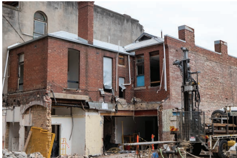
▲ The construction site at 364-370 Albert St, East Melbourne.
